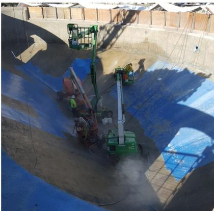
To begin, Thomarios performed high pressure water blasting at 40,000 psi. This surface preparation method was employed to completely remove the old coating and roughen up the underlying concrete to achieve a substrate suitable for mortar application.
