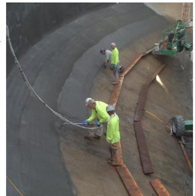
one pool presented a unique problem. The walls sloped at a steep angle down to the floor and made accessing these areas very difficult. To solve this problem, Thomarios temporarily attached plywood boards to the walls to stand on while applying the mortar. The ML-72P Mortar was then smoothed and finished.
