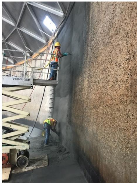
Mainstay ML-72 mortar was applied in 6-foot-wide sections at 1.5" thick using Madewell shotcrete equipment and scissor lifts. Each section was dampened with water prior to mortar application. The mortar was hand troweled smooth and broom finished to achieve a slightly textured surface. After finishing, a water-based concrete sealer was applied to prevent cracking.
