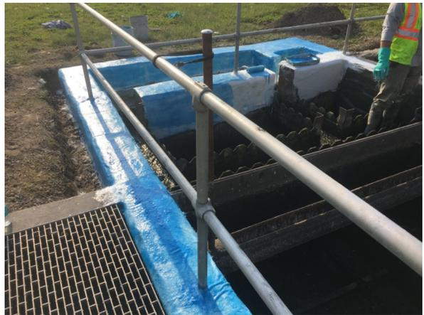
Culy's crew came back the next day to apply Madewell 927 Penetrating Epoxy Primer to the cured mortar. The primer was allowed to tack, and the crew applied a thin coat of Mainstay DS-5 100% Solids Epoxy Coating. The fiberglass reinforcement was then installed using fiberglass mat and cloth laid onto the wet epoxy and saturated with Madewell 1312E Epoxy Saturant. The material was left to cure overnight.
