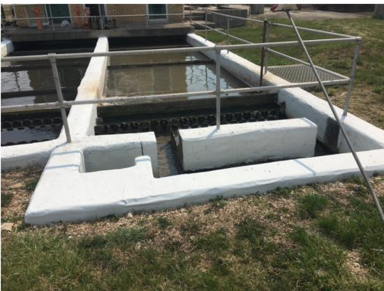
Upon returning the next day, the crew sanded the fiberglass layer to prep the surface for an epoxy topcoat and to remove any fiberglass strands sticking up from the surface. Lastly, a topcoat of Mainstay DS-5 Epoxy was applied to seal the fiberglass system, provide a smooth, continuous surface, and prevent any future concrete deterioration.
