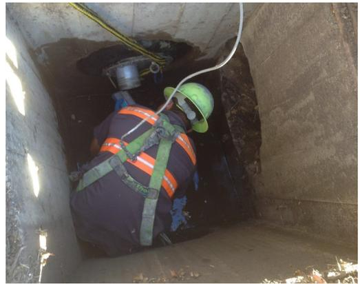
After cleaning, H&R Plumbing utilized Madewell's horizontal mortar spinner to centrifugally apply 3/4" of Mainstay ML-72 Restoration Mortar to the inside
